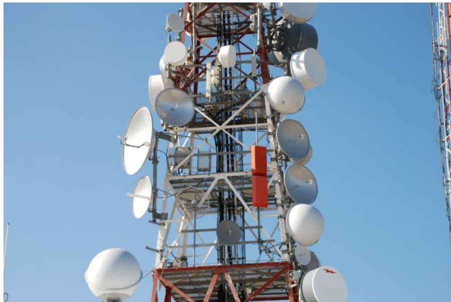
A variety of parabolic antennas on a communications tower in Australia for point-to-point microwave communication links
