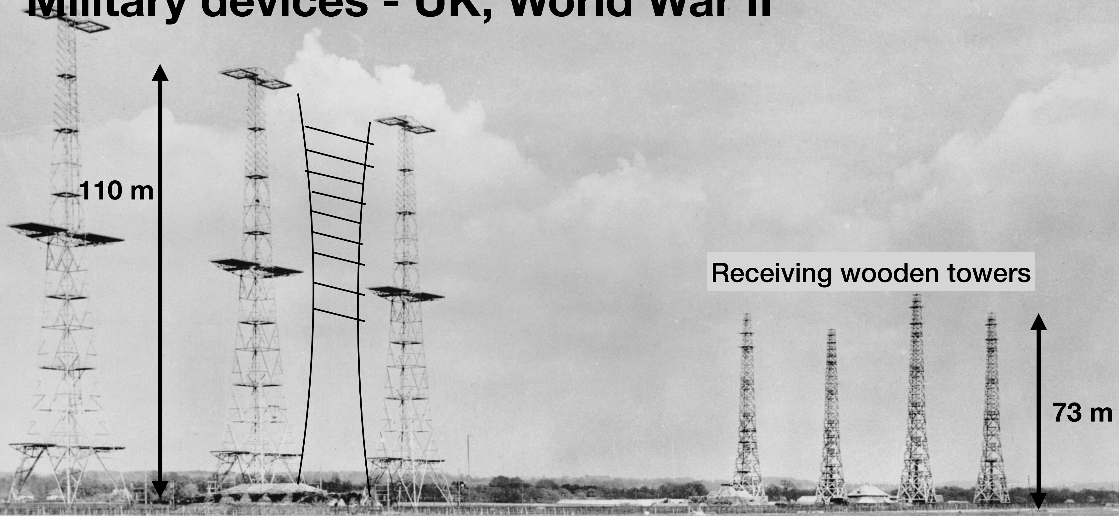
Transmission steel towers (4)
