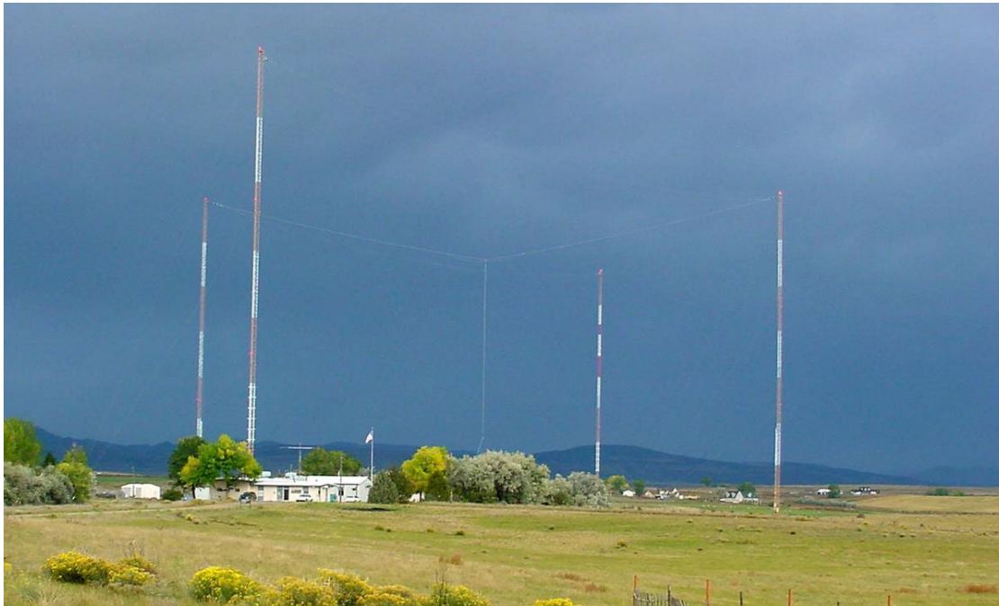
WWV Transmitter near Fort Collins, CO, [32]
