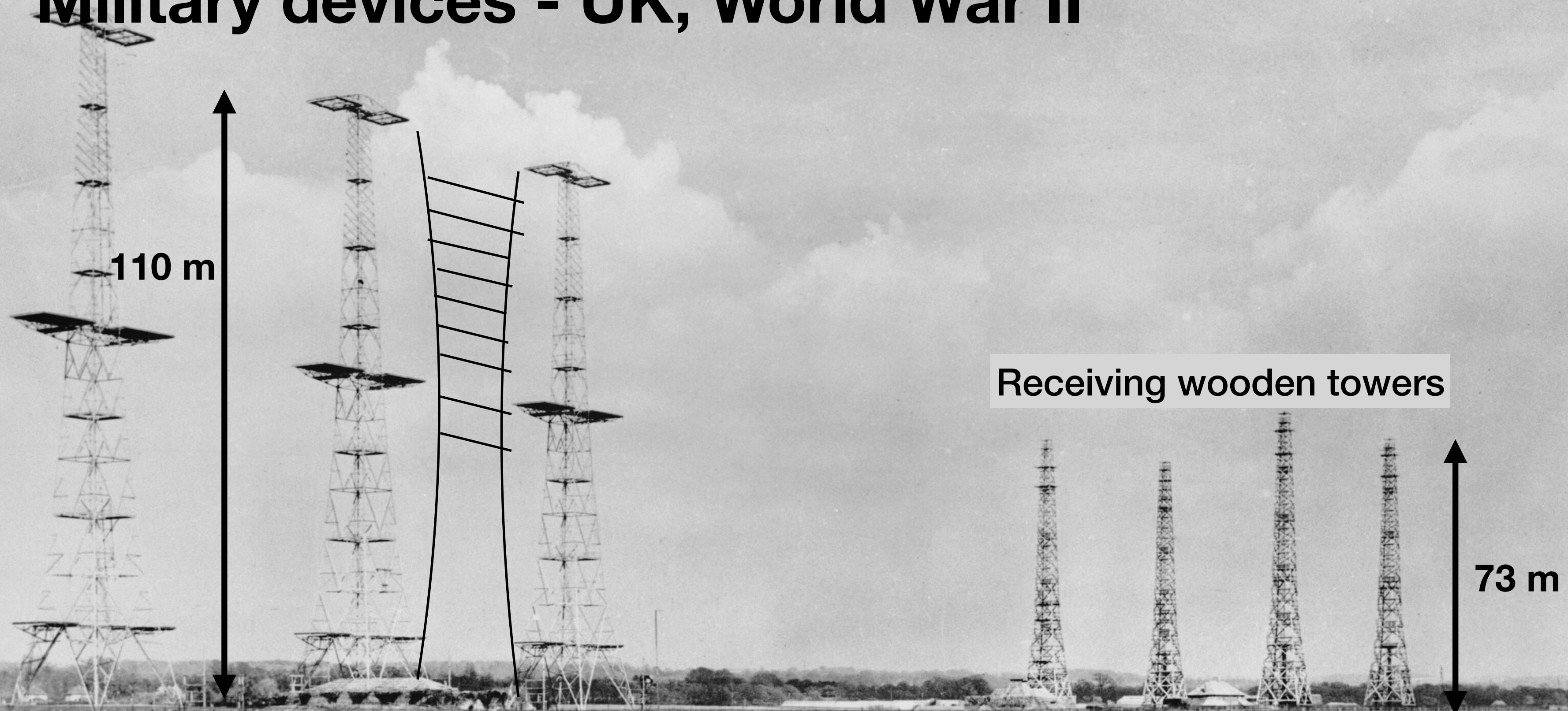
Transmission steel towers (4)
