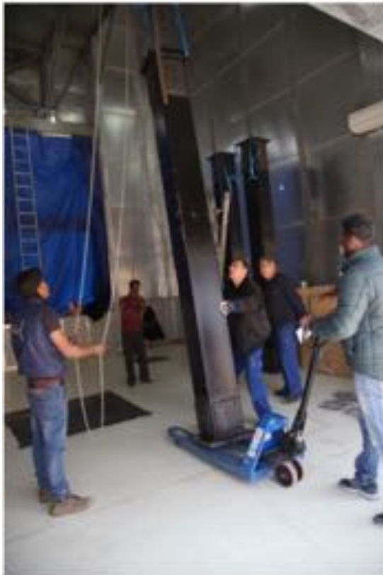
Erection of the ILMT structure on 4/3/2017.
