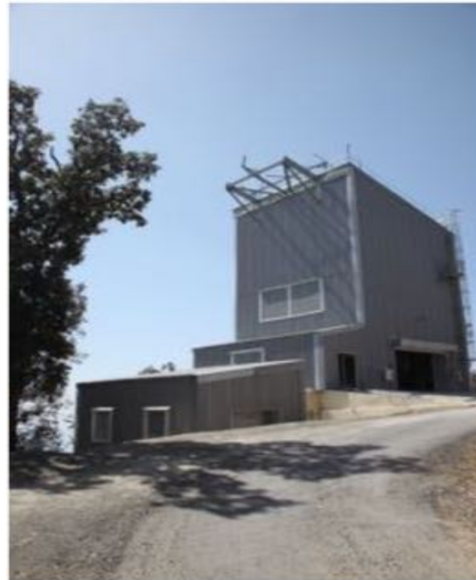
ILMT compressor, control and main ILMT buildings
